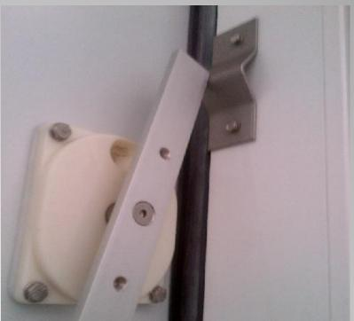
**Guaranteed airtightness** by means of double, high flexible co-extruded EPDM gasket.
