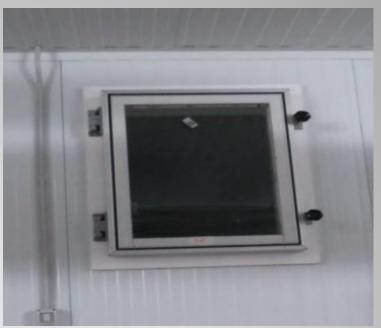
**800X600 Control window installed in the leaf.** Airtight closure by means of pressure wheels
